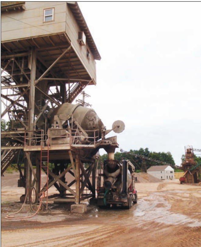
Figure 29. Central ready mix concrete plant in the process of lifting the batch mixer to load the wet mix into a transit mixer truck. Courtesy Northern Ready Mix, Inc.
