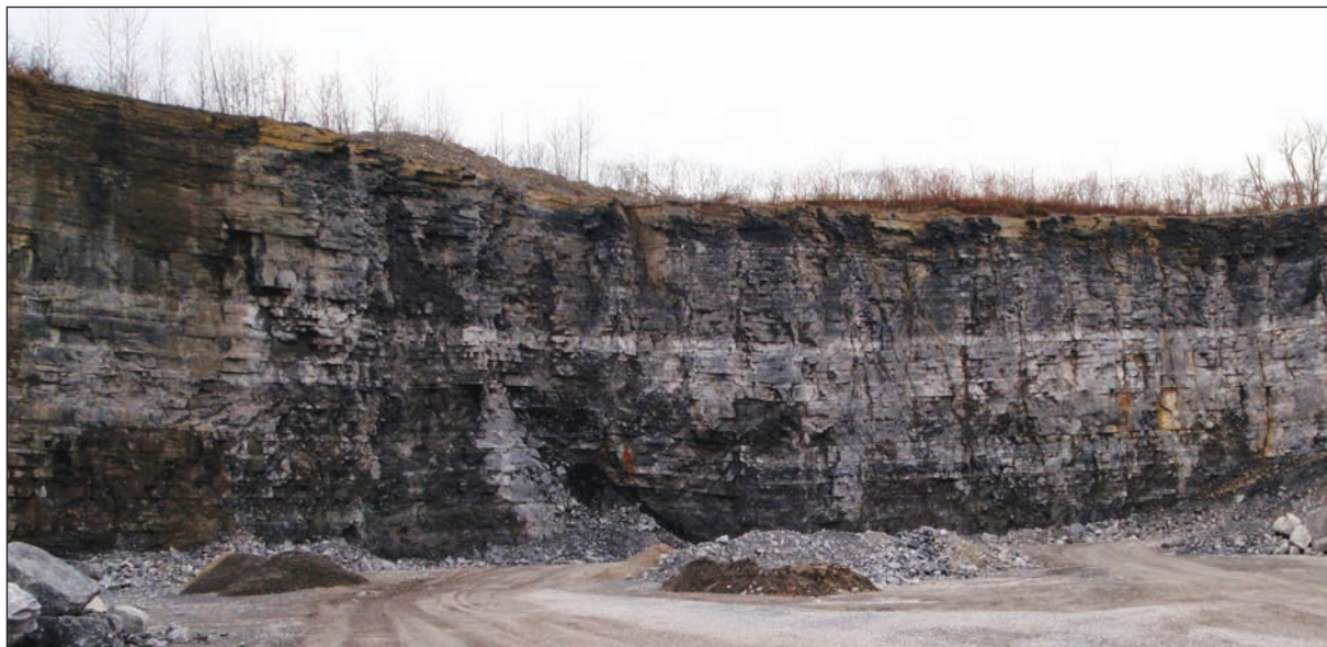
Figure 14. Quarry face in a carbonate rock quarry. The geological formations are nearly horizontal. Courtesy Callanan Industries, Inc.
